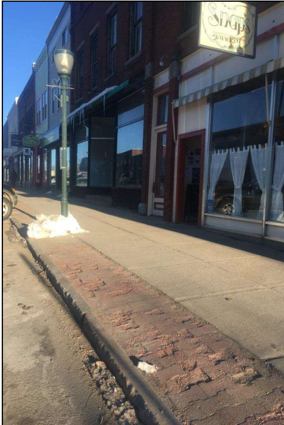
Figure 2. Deteriorated brick pavers, granite curbing, and lamp post buried in snow. (March 2018)
