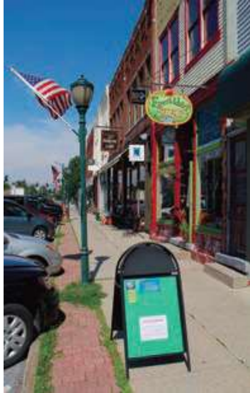
Figure 4. Existing worn, edge pavers to be replaced to match 2015 improvements. (2017)
